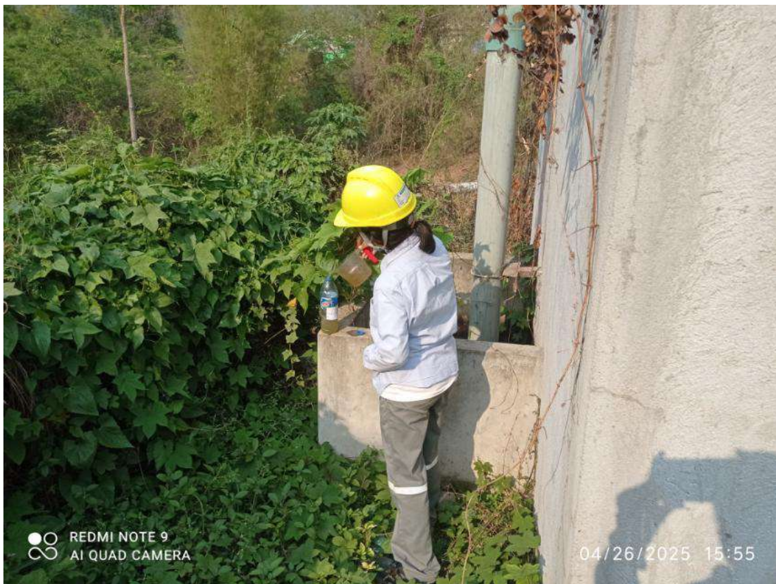
Bio tank Effluent
