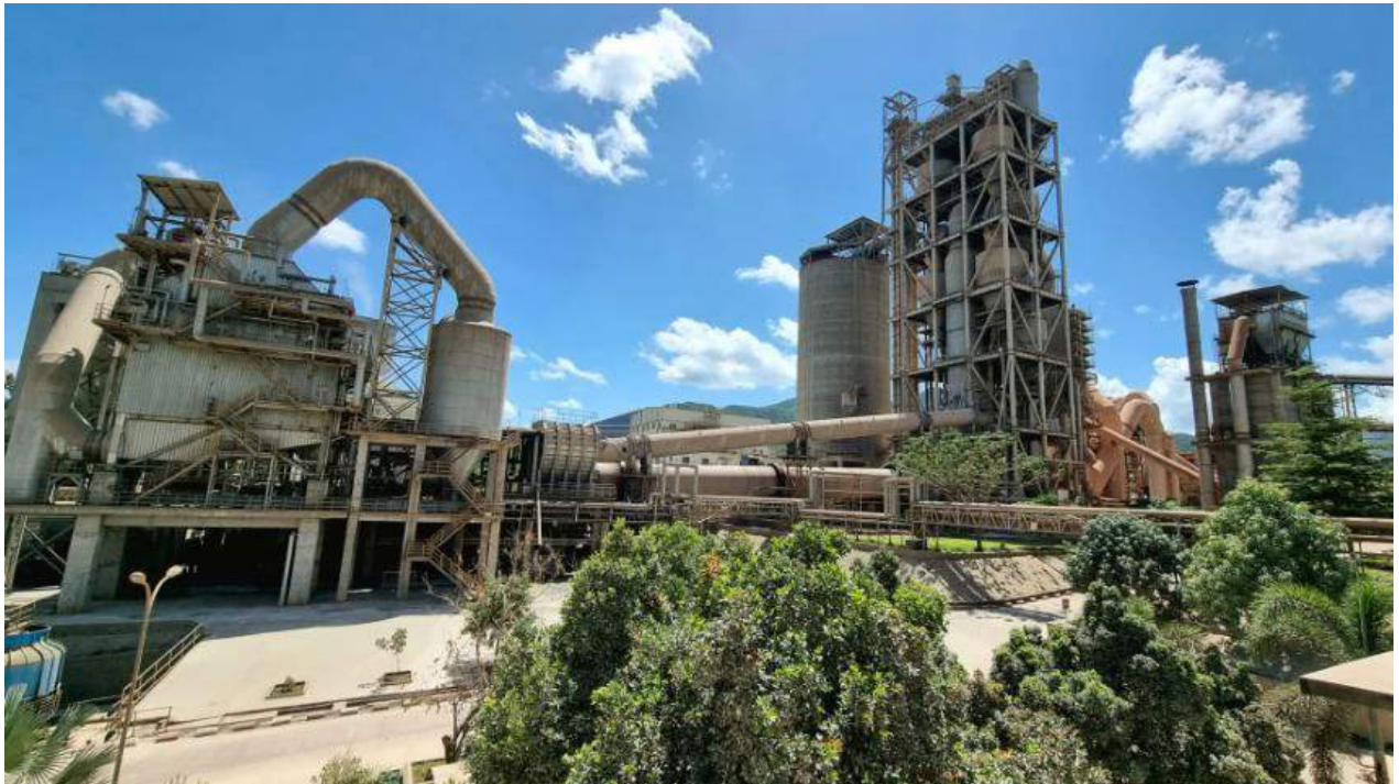
Figure 3. WHR System in STC Cement Plant
